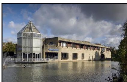
Stockley Park, Uxbridge Registered Grade II August 21 st 2020
